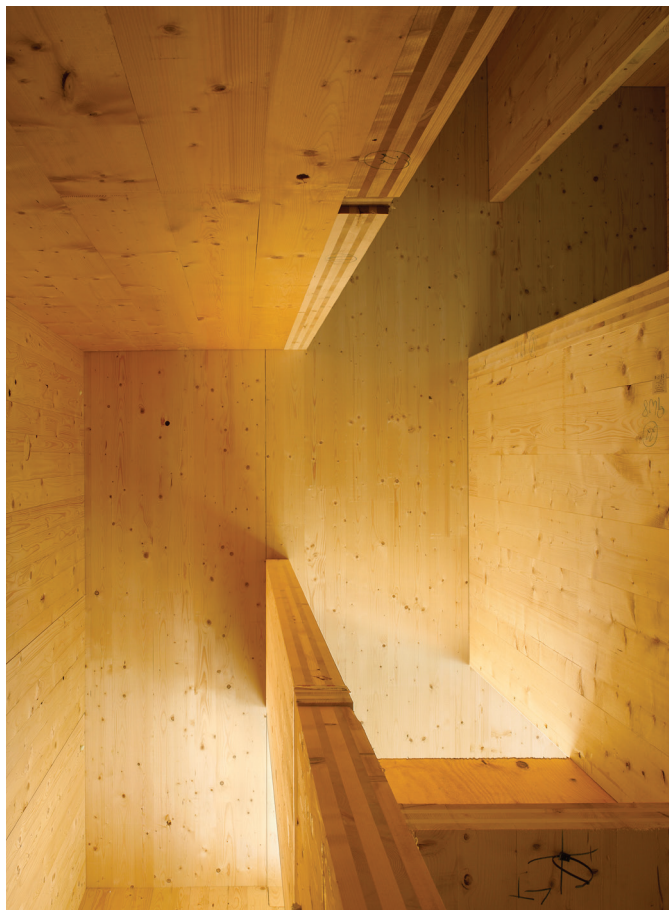
CLT walls and floors in Murray Grove
