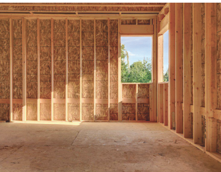
Lightweight timber frame with OSB sheathing
