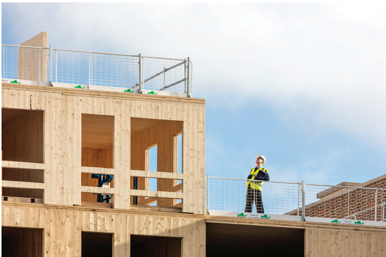
CLT external walls with pre-formed fall protection and window openings, Dalston Works
